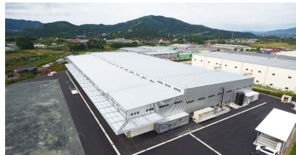
Shinshiro factory Site area : approx. 27,000 m 2
