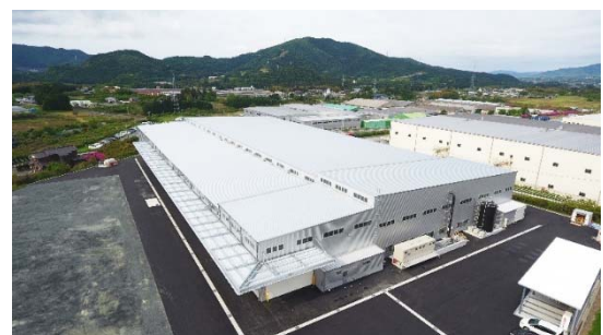
Shinshiro Plant Site area: approx. 27,000 m 2
